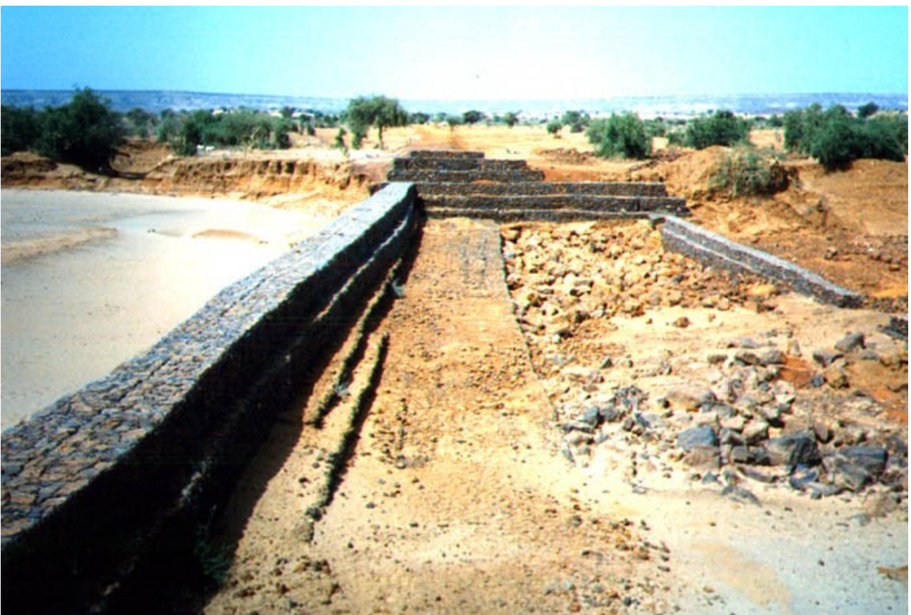
Fig. 1.2 - Gabions weir
