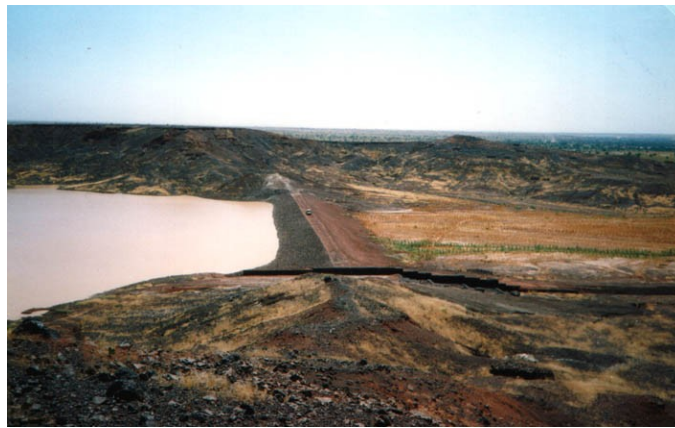
B – side spillway
