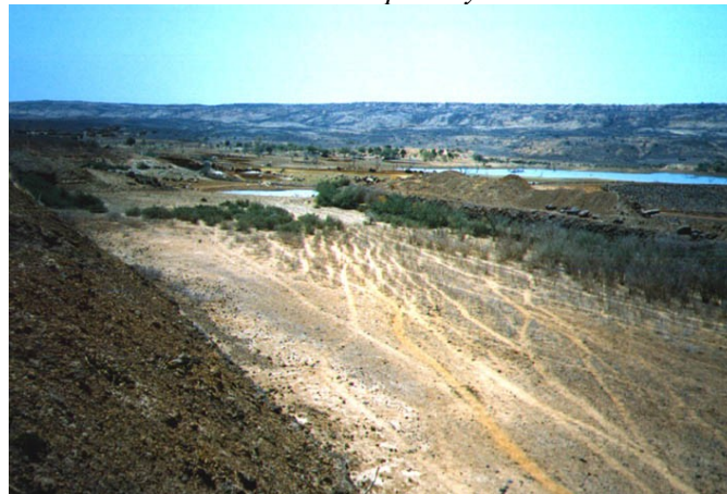
B – lateral spillway
