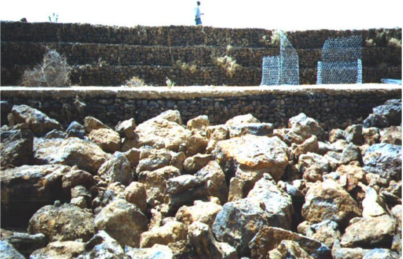
Fig. 4.27 – Lining of stilling basin with blocks
