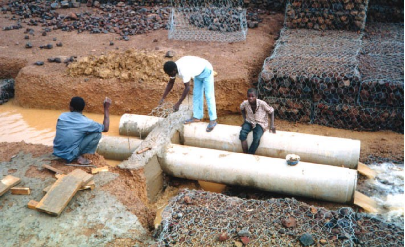
Fig. 4.10 – Cut-off collars preparation
