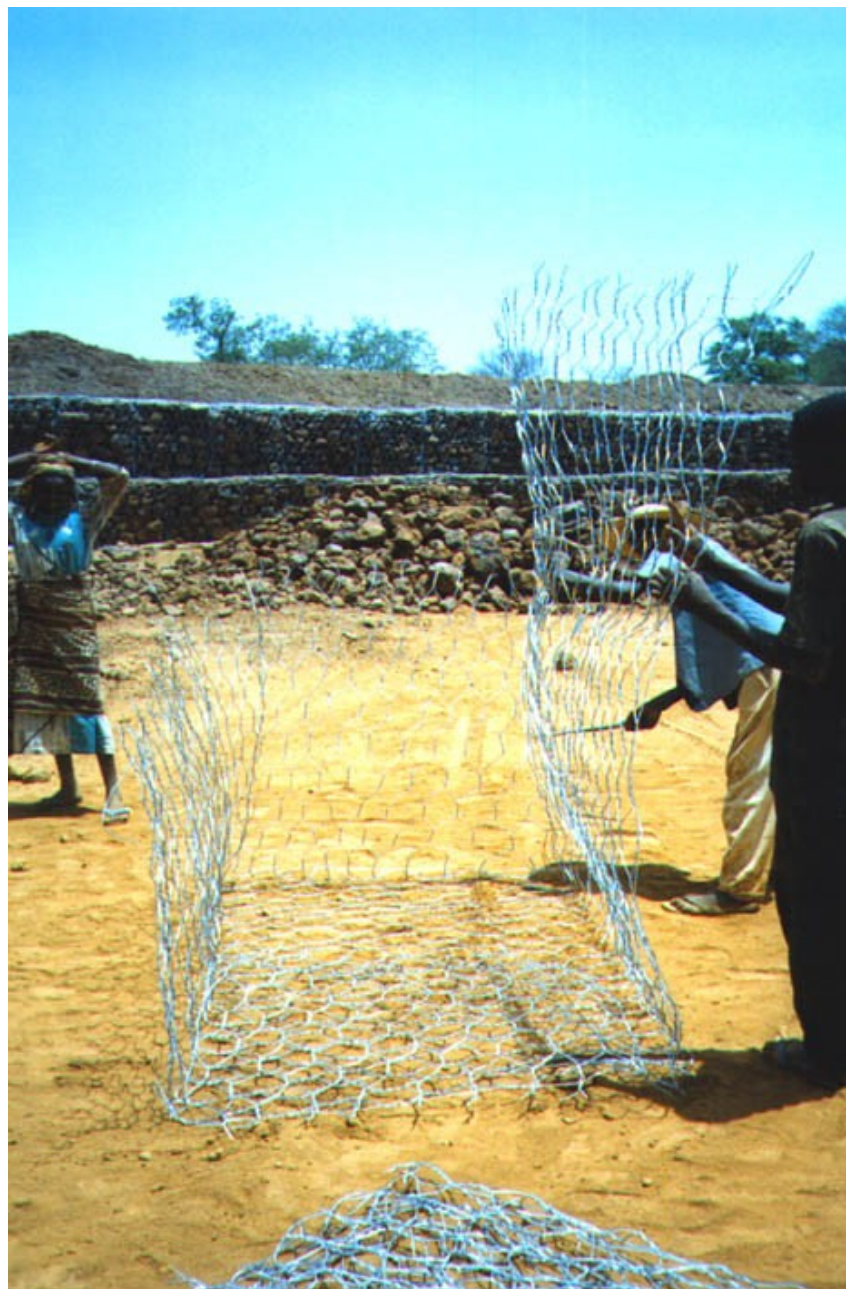
Fig. 4.20 – Gabions basket assembling
