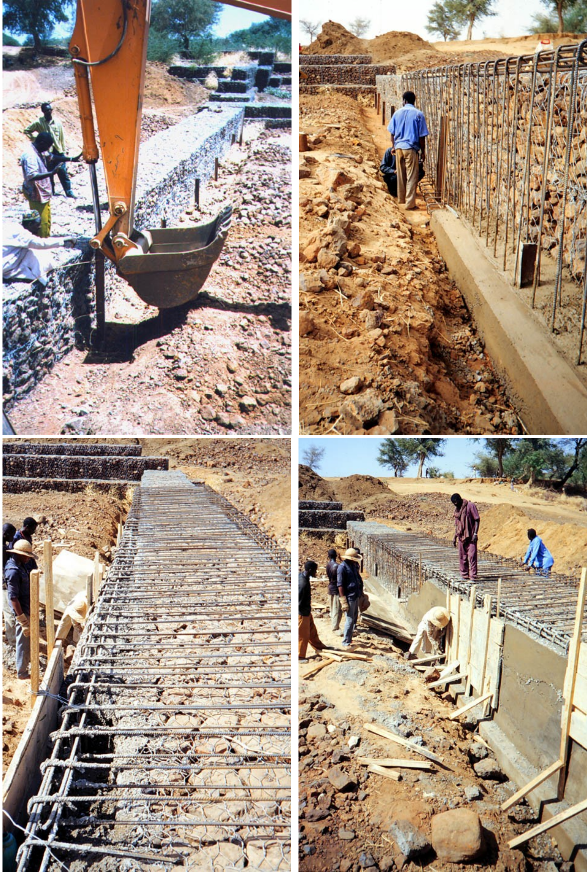
Fig. 4.31- Lining and anchoring a counterweir, Keita's Valley in Niger, 1999.
