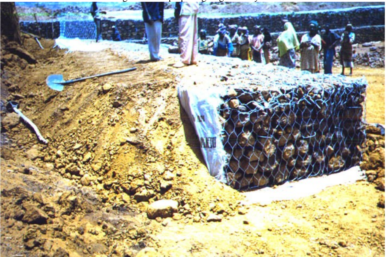
Fig. 4.24 – Fill compaction next to the gabion
