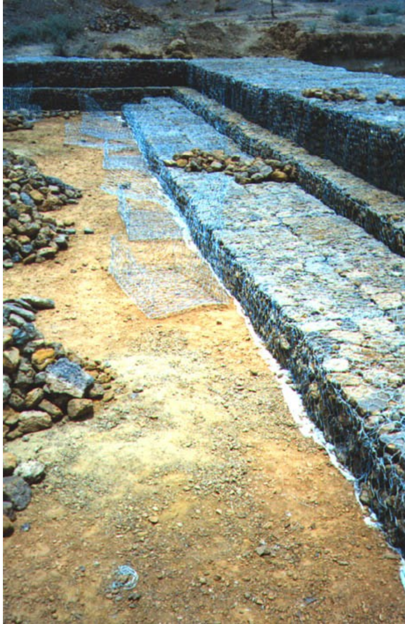
Fig. 4.21 – Gabions positioning
