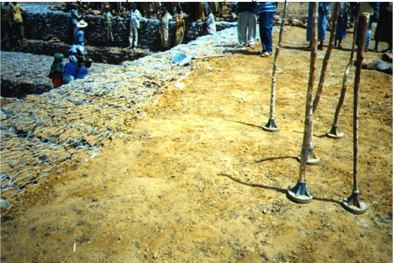
Fig 4.16 – Manually compacted layer
