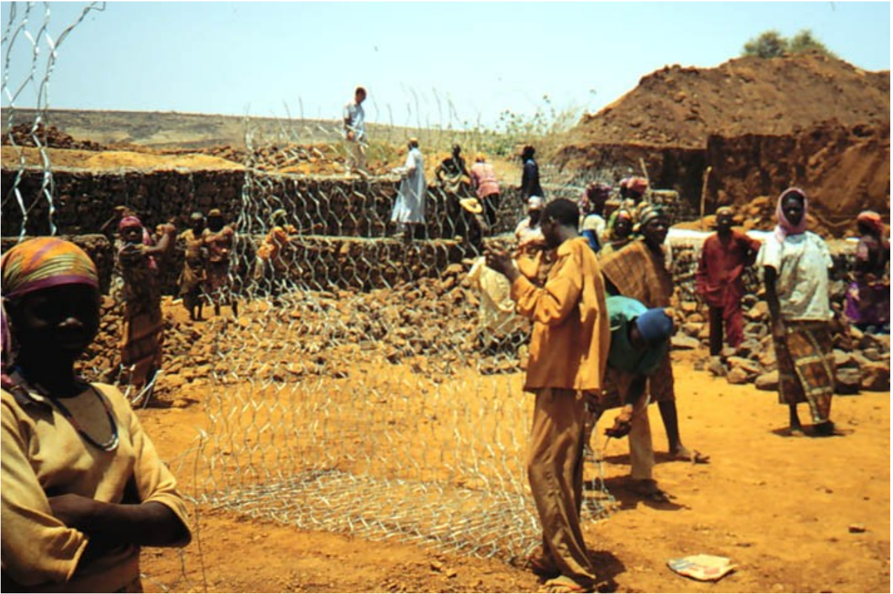
Fig. 4.19 – Gabions net opening
