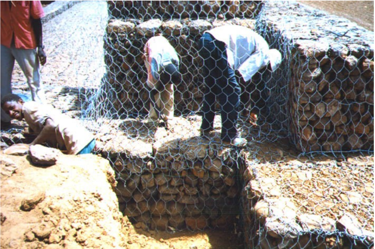
Fig. 4.23 – Superposing of gabion layers
