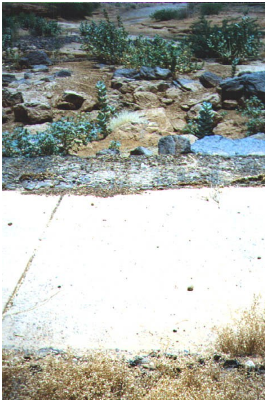
Fig. 4.29 – Lining of stilling basin with slabs of reinforced concrete
