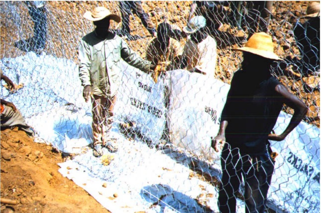
Fig. 4.32 – Semi-permeable cut-off screens
