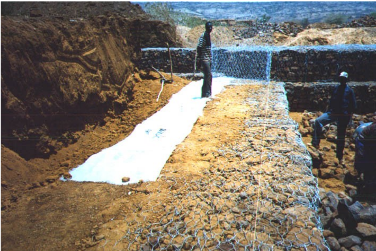
Fig. 4.17 – Placement of geotextile
