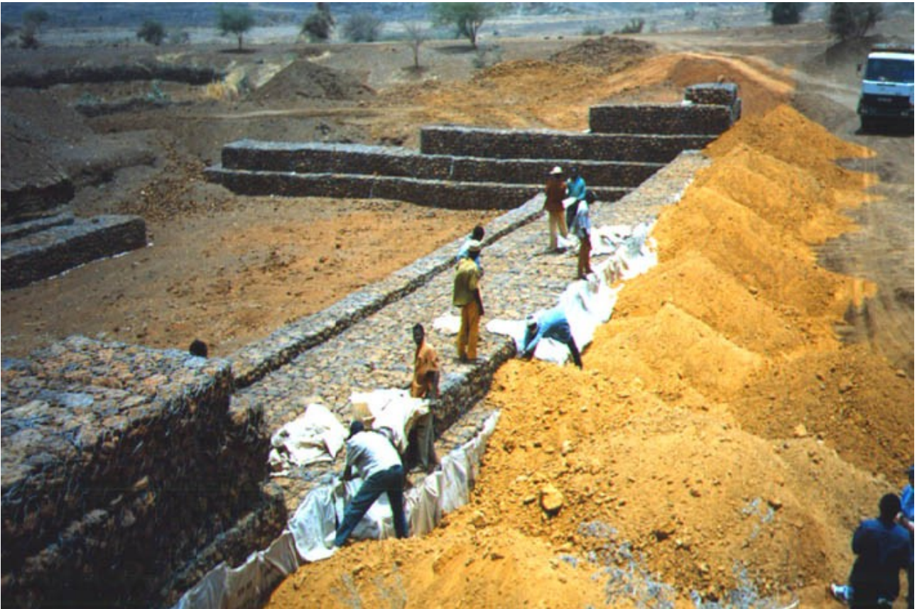
Fig. 4.25 – Earthfill used to waterproof the weir
