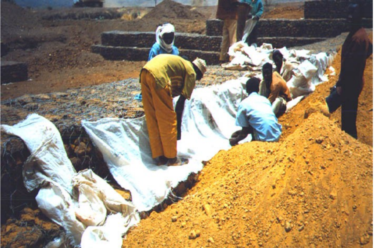
Fig 4.26 – Geotextile placement
